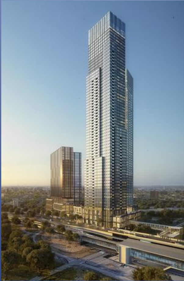
Trinity Centre at Bayview
